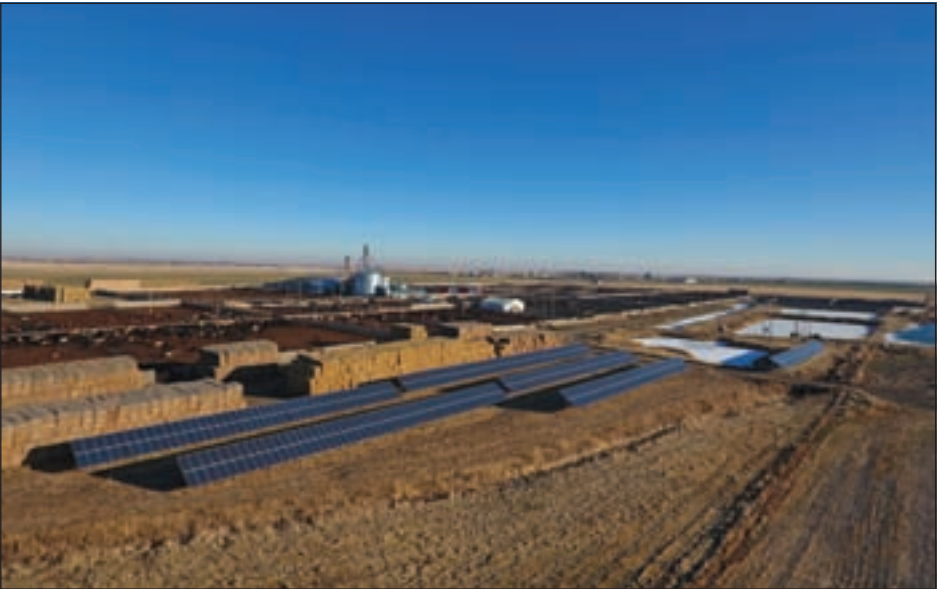
The 200-kilowatt array on Nelson Family Ranches is big enough to supply electricity to both its feedlot operation and irrigation pivots. PHOTO: NELSON FAMILY RANCHES
