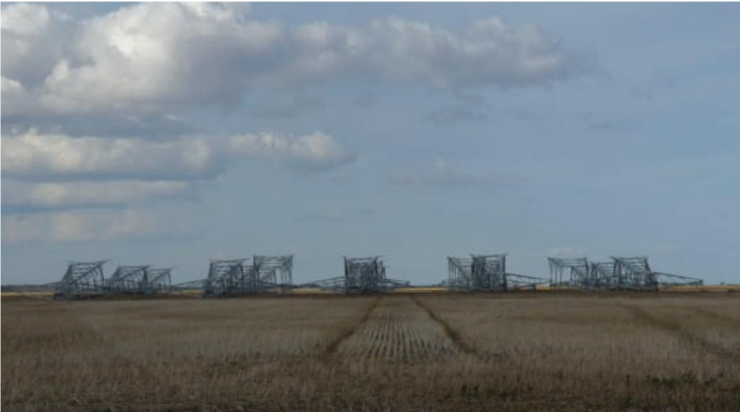
These tower tops for the new Bipole III line await lifting into place. PHOTO: SANDI KNIGHT
