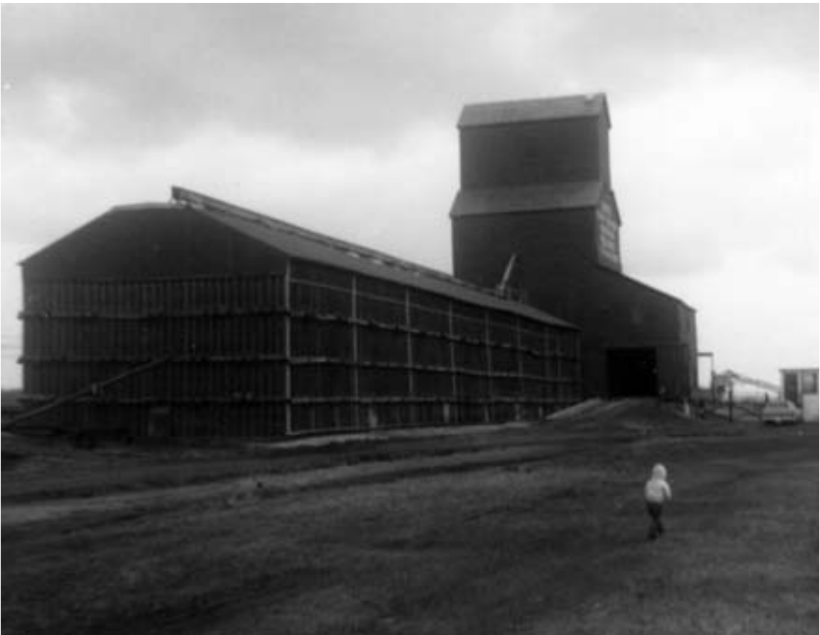
A 30,000-bushel wooden grain elevator at Curtis, in the Rural Municipality of Portage la Prairie, was built in 1938 by Portage businessman Andy Forsythe. His Forsythe Elevator Company was one of the first companies west of Winnipeg to use grain-drying equipment. He introduced a fairer method for determining dockage, and successfully challenged the Canadian Pacific Railway over its blockage of highway rights-of-way, resulting in revised railway practices that are still in place today. Sold to Reliance Grain in 1946, the Curtis elevator was resold to Manitoba Pool in 1948 and a large balloon annex was built beside it in 1951. The elevator closed in July 1972 and was removed from the site. PHOTO: UNIVERSITY OF MANITOBA ARCHIVES & SPECIAL COLLECTIONS
