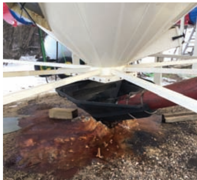
When the high-moisture canola that caused the gate to freeze shut was finally melted, it released what Bown called "canola juice" out the bottom of the bin.
