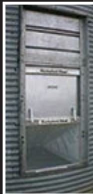
Tie bar bolts on with wing bolts.
